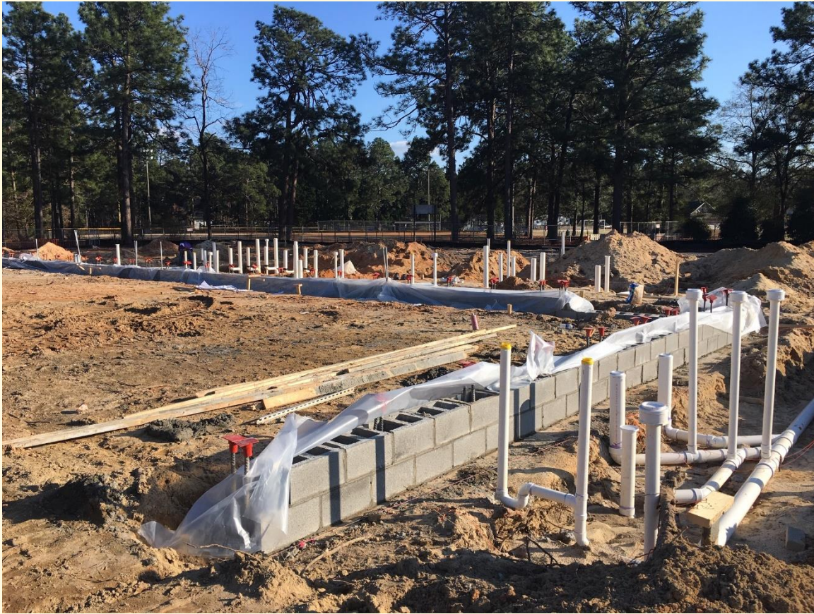
Underground Plumbing/Electrical
